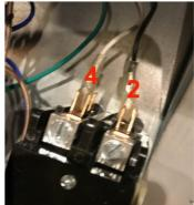
Below is The Single Throw relay (contactor) that we use to replace the OEM contactor.
